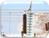
송배전 / 비행시설 Electric Power Supply / Air field
